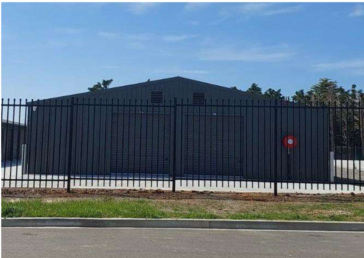
New buildings in Red Fields Road
